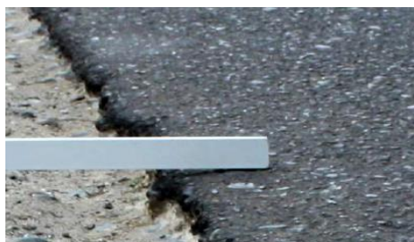
Figura 13. Desnivel Carril / Berma (m)
