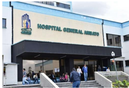
Figura 1.15: Hospital General Ambato IESS [20].
