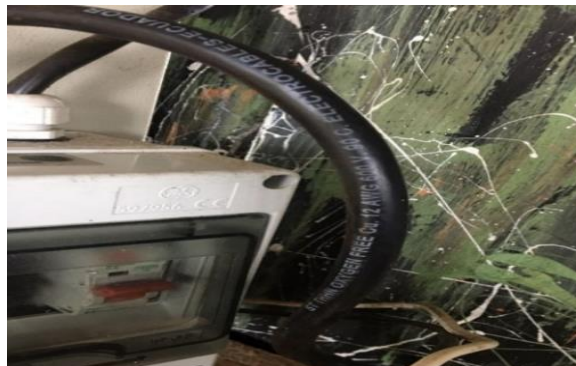
Figura 3-14: Conductor multipolar ST-THHN.
