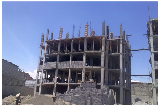
Columnas H 0 E 0 f c =210 kg/cm 2
