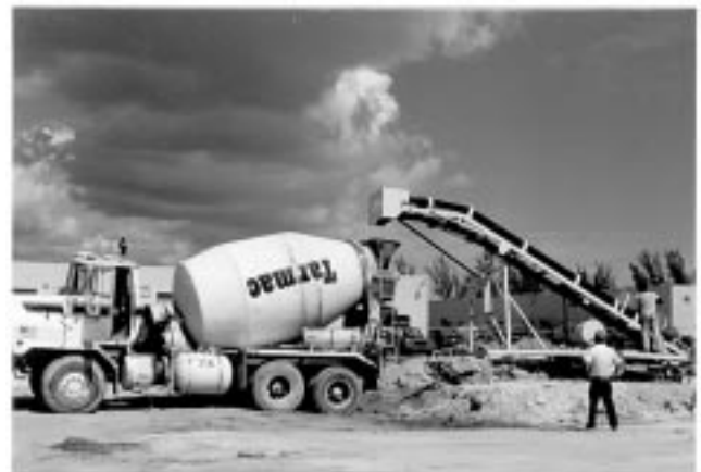
Fig. 2.7—Adding steel fibers to a loaded mixer truck via conveyor
