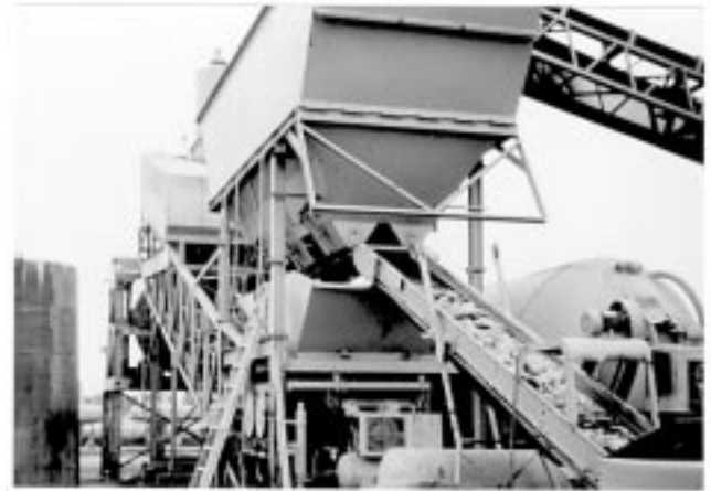
Fig. 2.9—Adding steel fibers to weigh batcher via conveyor belt
