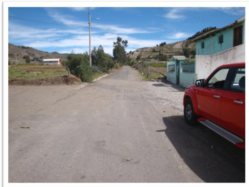
Chilla Grande Km 7+473.92
