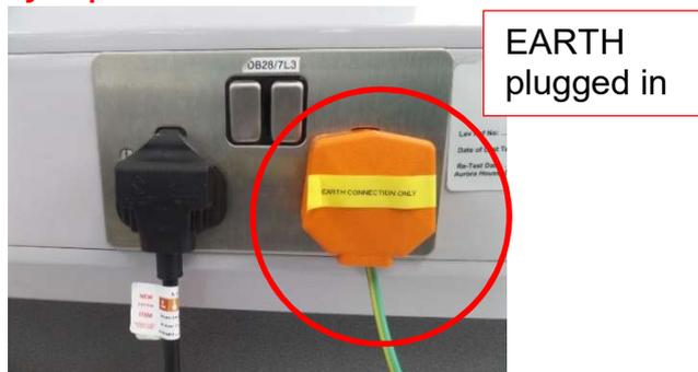
Figure 4: EARTH lead is plugged into mains
