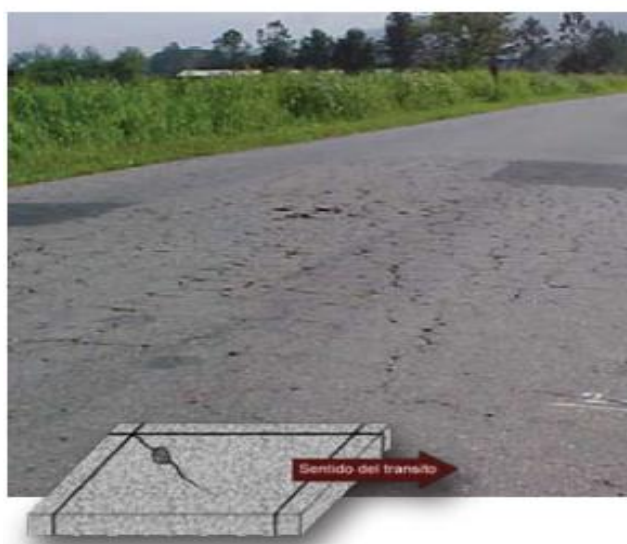
Figura 1. 25: Fisura Inducida [31].
