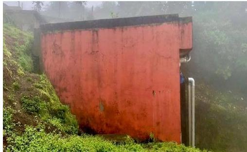
**Figura 15:** Tanque IMHOFF (PTAR).
