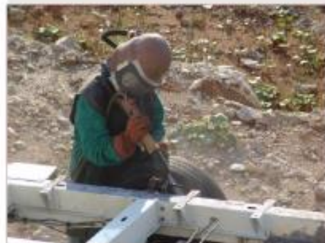
Example of sandblasting with garnet:
