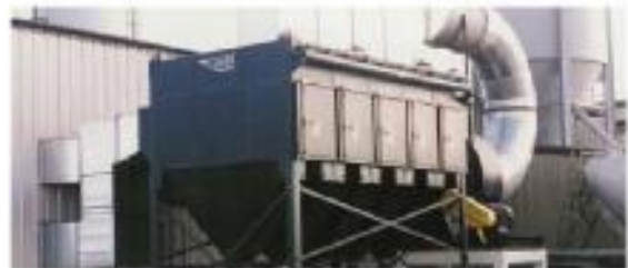
GS 50 on Sand Blasting
